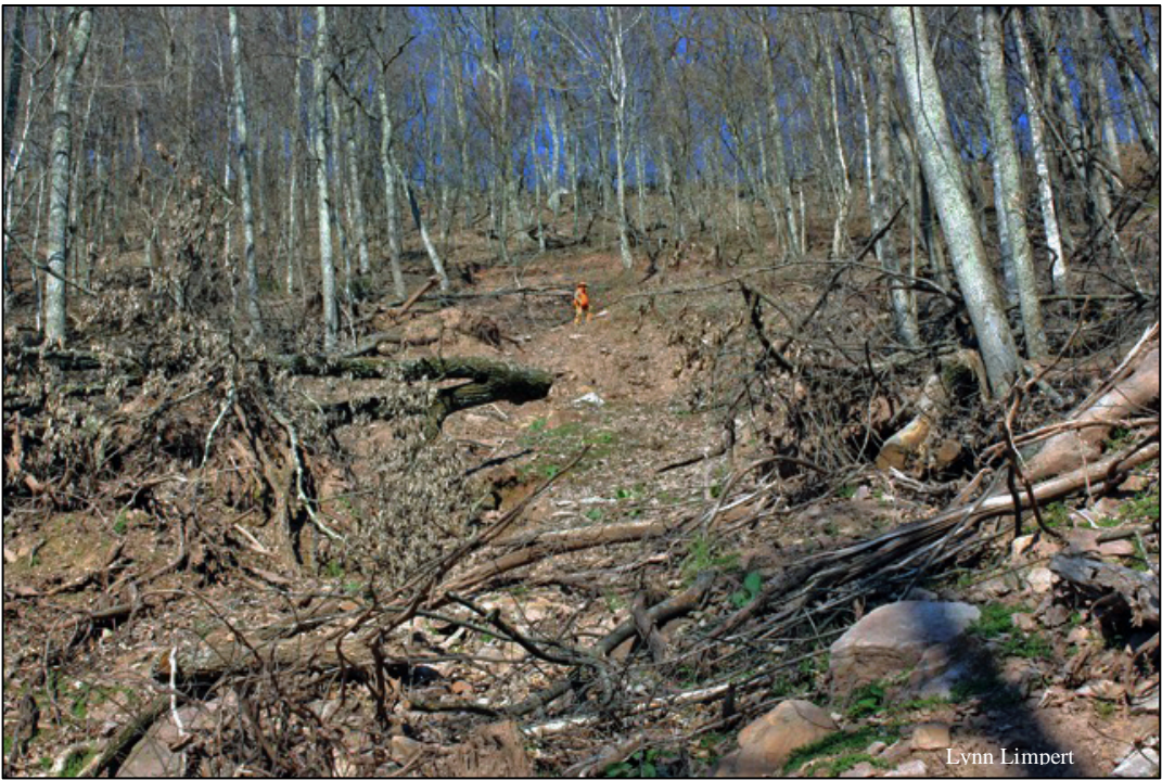
Figure 4 400-foot landslide on a 62% slope near the top of Little Mountain below the proposed ACP corridor.
