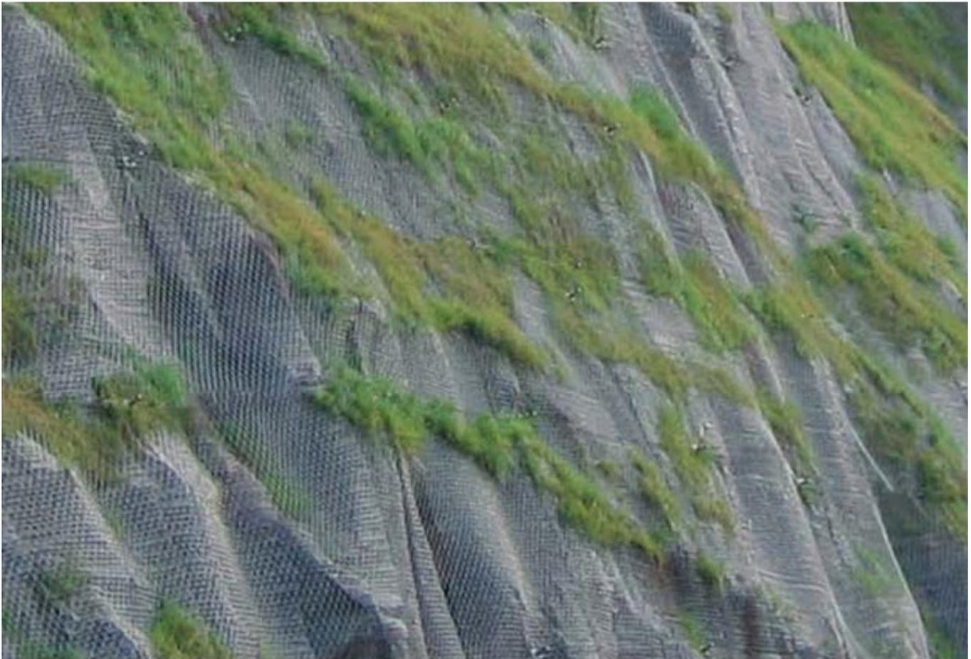
Steel-wire mesh similar to that proposed for use on steep slopes along the Atlantic Coast Pipeline corridor.
