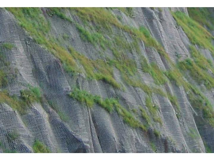
Steel-wire mesh similar to that proposed for use on steep slopes along the Atlantic Coast Pipeline corridor.
