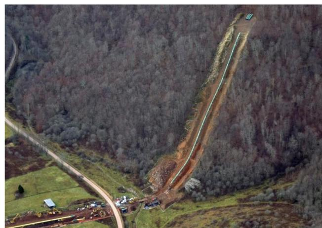
ACP CONSTRUCTION IN POCAHONTAS COUNTY. WATER BARS ARE NOT INSTALLED AS REQUIRED FOR STEEP SLOPE CONSTRUCTION.
